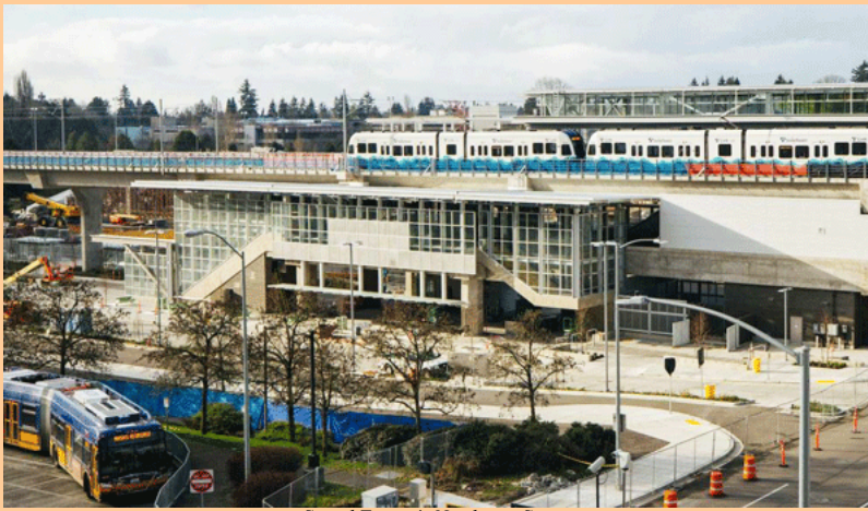
Sound Transit's Northgate Station
